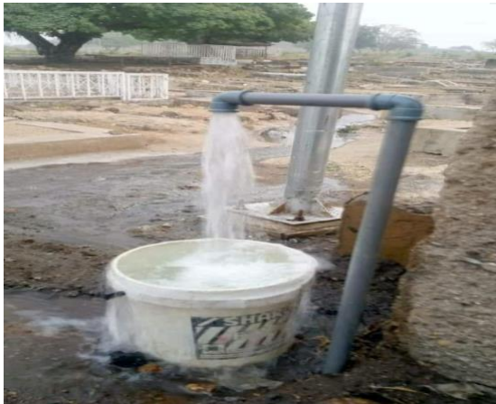
Construction of Industrial Borehole in Okene cemetery
